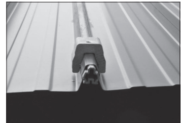
Example of correctly installed S-5-KHD clamp
